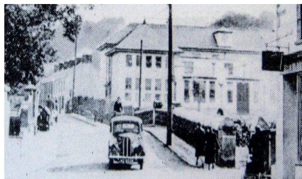
Picture of the bridge over the Inver River with Larne and Inver PS in the background: 1940s
