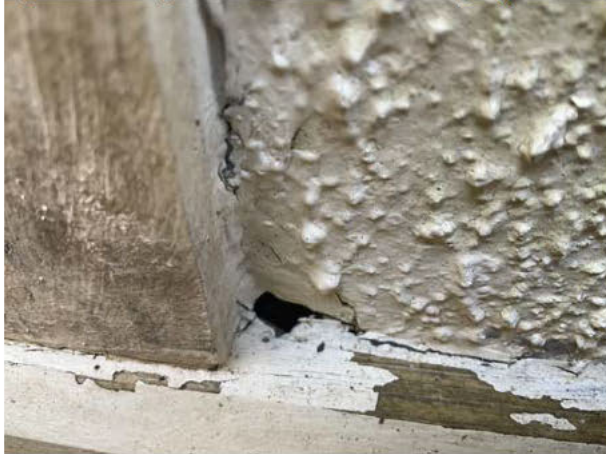
Figure 112.10 (southeast elevation underneath middle window)
