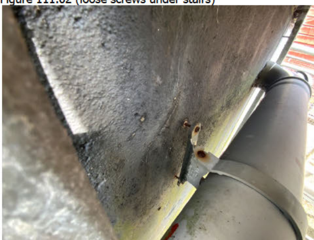
Figure 111.02 (loose screws under stairs)
