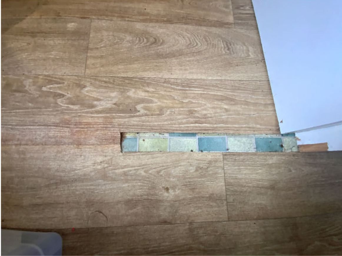
Figure 115.03 – previous vinyl flooring covered with newer wood effect vinyl flooring
