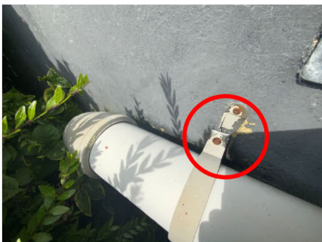
Figure 111.02 (loose screws under stairs)
