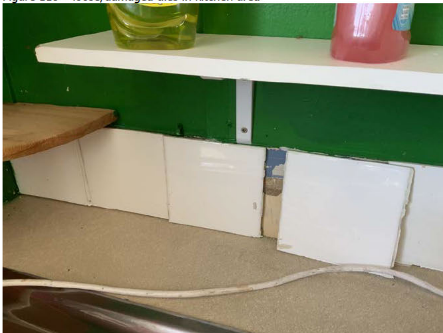
Figure 118 – loose/damaged tiles in kitchen area
