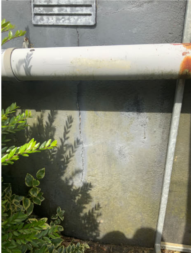
Figure 110.01 (southeast elevation behind loose downpipe)
