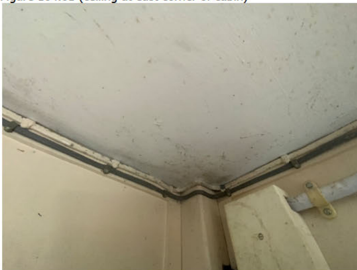
Figure 104.02 (ceiling above main entrance door)
