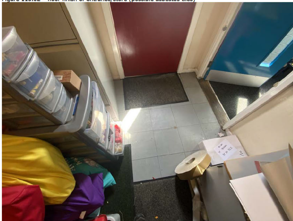
Figure 115.02 – floor finish of entrance/store (possible asbestos tiles)
