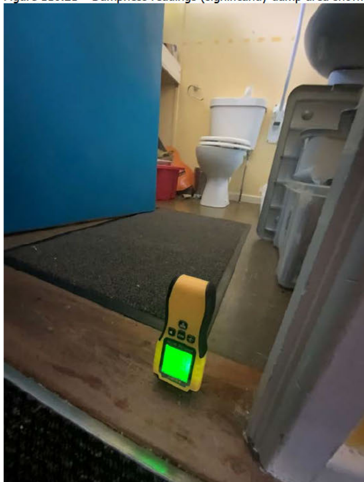
Figure 116.21 – Dampness readings (significantly damp area shown here for door saddles)
