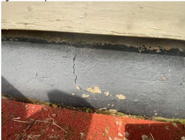
Figure 110.07 (southeast elevation underneath middle window)
