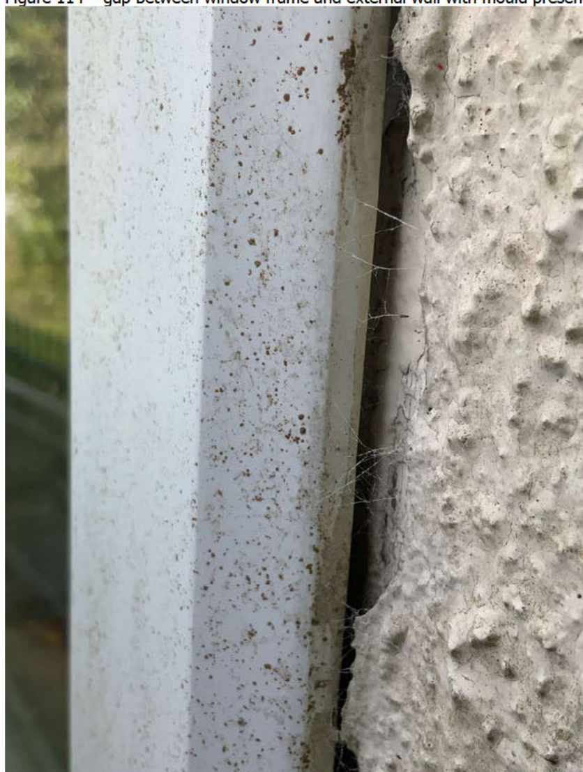
Figure 114 – gap between window frame and external wall with mould present
