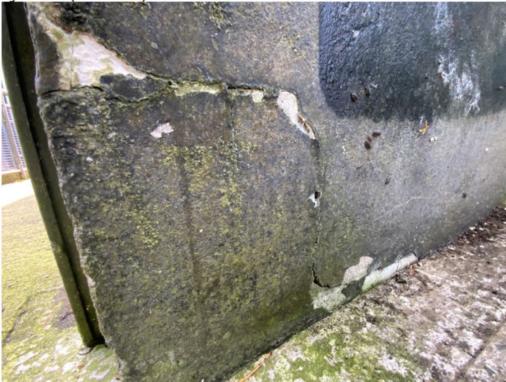
Figure 110.06 (southeast elevation beside gully)
